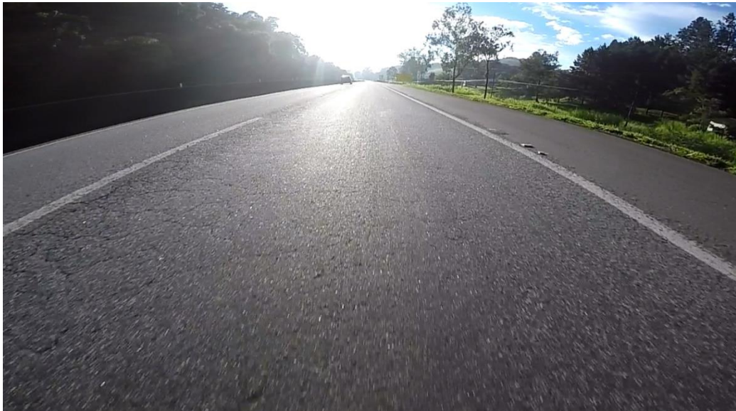
Figura 144 – Trecho experimental 03 (TE-03, km 708+450 ao km 708+850, UF: MG)
