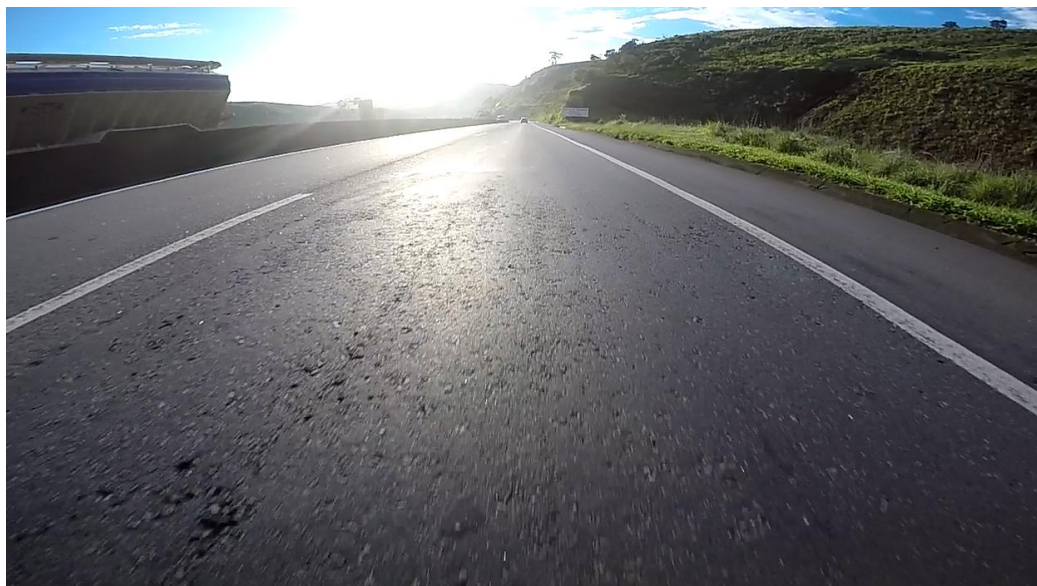
Figura 147 – Trecho experimental 04 (TE-04, km 728+300 ao km 728+700, UF: MG)
